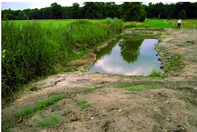
Fig. 9: View in flow direction of the „Sediment trap Bargfeld“ in summer of 1999 about one year after completion and after the first time of excavation. In front of the left side the mouth of the drainage ditch can be seen. At the far end on the left of the sediment trap the drainage ditch continues its flow through dense vegetation.
